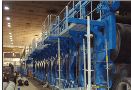
ARC S1 applied to frame during refurbishment
